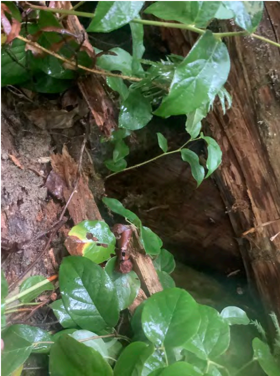
Right Bank Abutment when facing downstream
