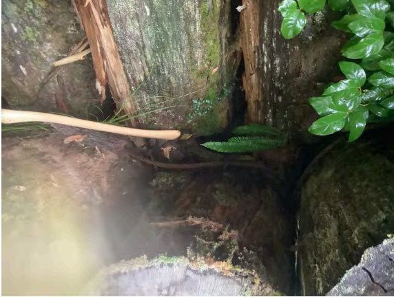
Right Bank Abutment when facing downstream - tiebacks in fair condition
