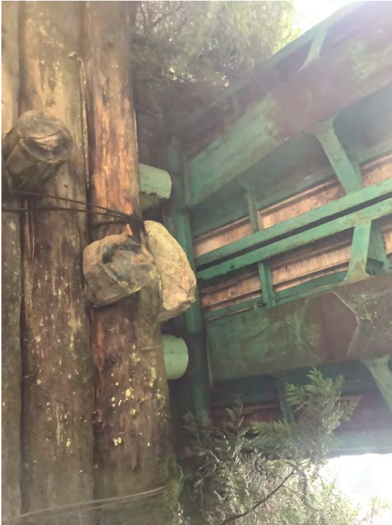
Right Bank Abutment when facing downstream
