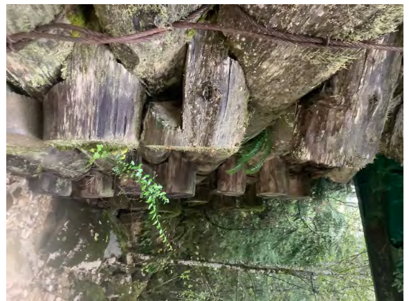
Right Bank Abutment when facing downstream
