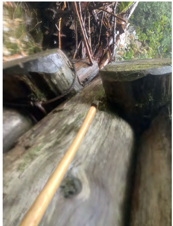
Right Bank Abutment when facing downstream
